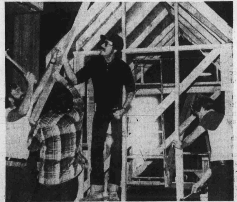
SANTA'S HOUSE UNDER CONSTRUCTION - The Henderson Rotary Club, aided by Lt. Jim Thompson of the Salvation Army, is constructing a house for Santa Claus. Pictured working on the house are, from left: Lt. Thompson, Gary Johnson, Bill Perry and John Holman.
