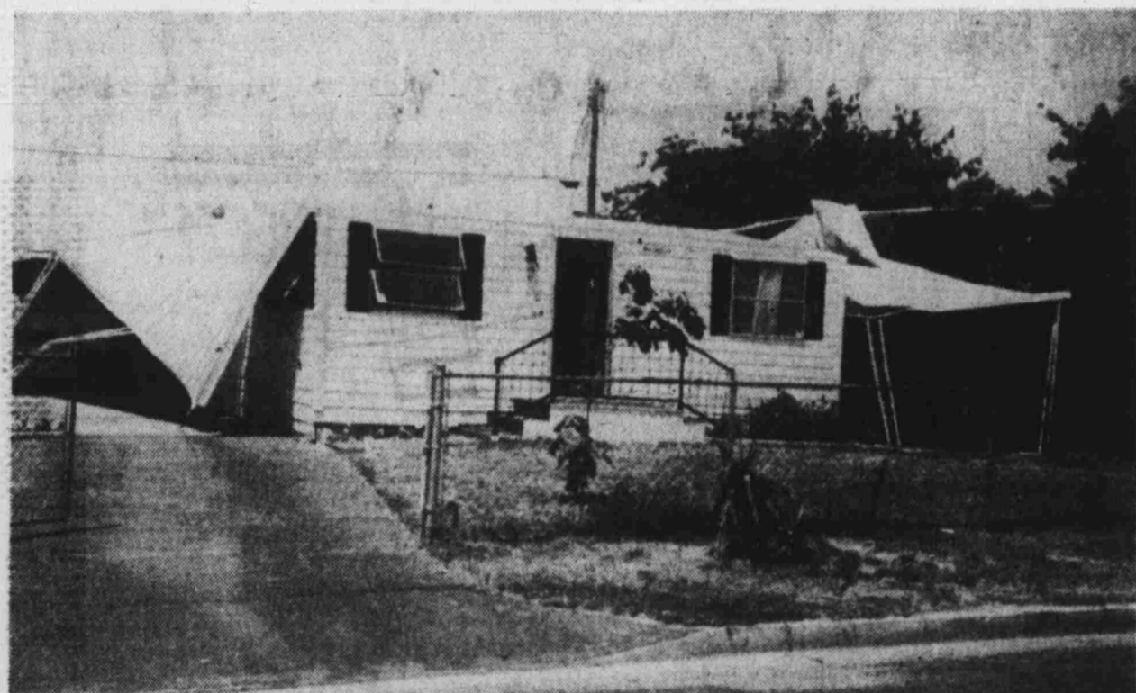
DUSTER TAKES ROOF-Last Friday a not so friendly wind duster removed the roof from the trailer home of Mr. and Mrs. Erwin Peders who live in Henderson
