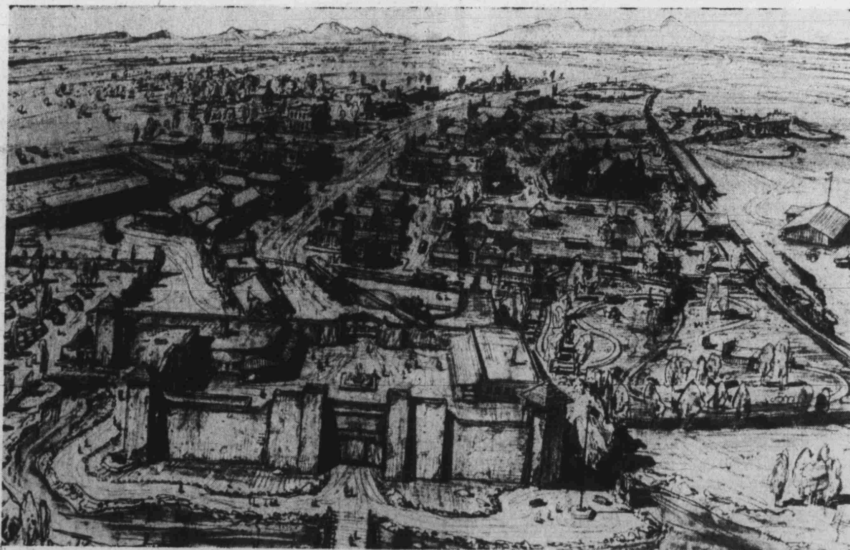
OLD VEGAS CONSTRUCTION -- Old Vegas, a family oriented western theme park depicting the colorful history of Southern Nevada, is now under construction on the Boulder Highway south of Hen-
